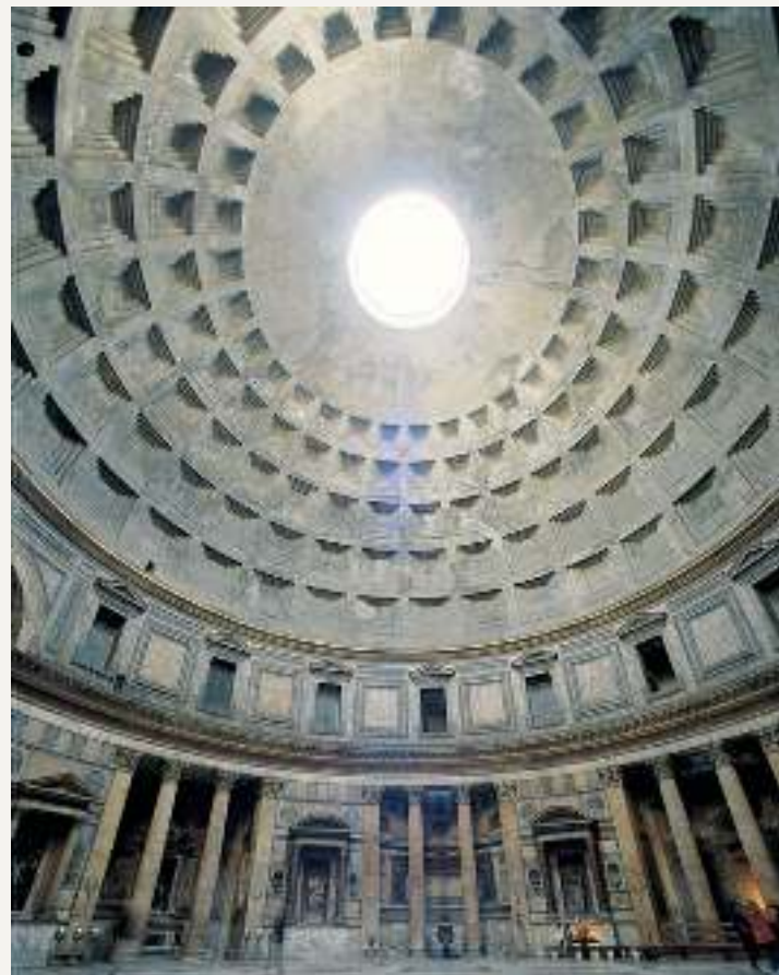
Roman dome with oculus (Pantheon, Rome, Italy, 118–125)
