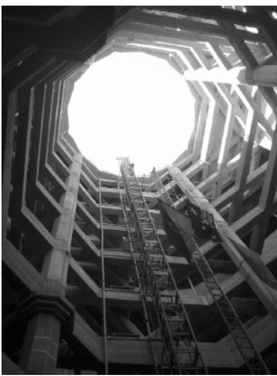
Open shaft at the centre of the Flats.
