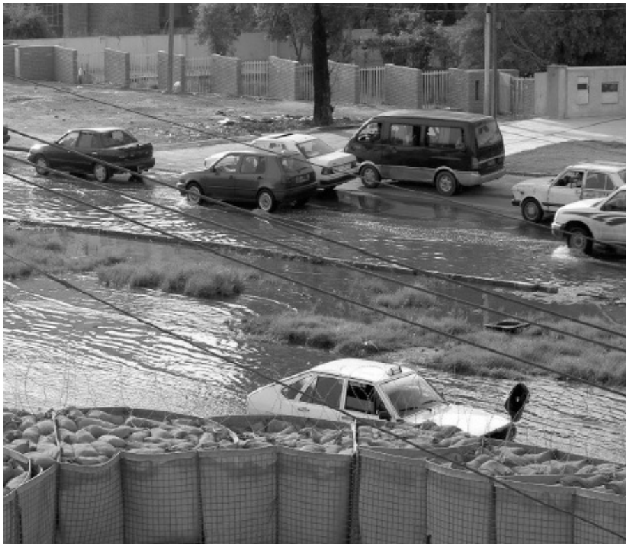
Streets of Baghdad with overflowing sewage.
